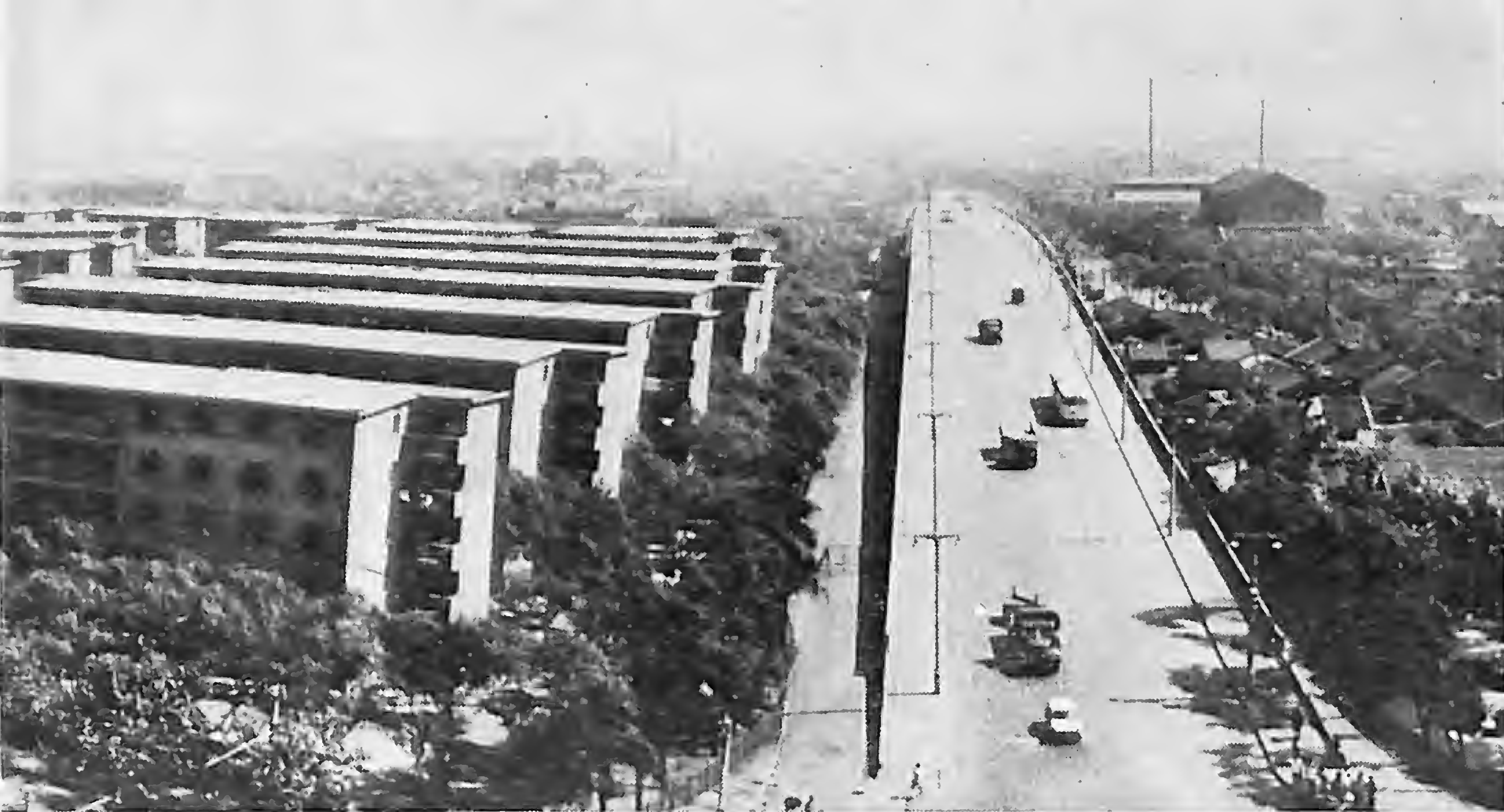
The new workers' village on Melon Lane, Shanghai.
